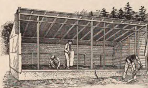
Fig. 569. Interior of hen-house in process of construction. Finished structure shown in Fig. 555.
